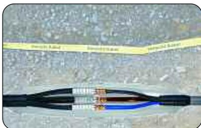
The procedure for the copper section is absolutely identical as on copper compression cable lugs. The crimping marks on the product give detailed information as to origin and application of the Al/Cu compression joints. The marking "KL14 50 rm/70 re/se" signifies
