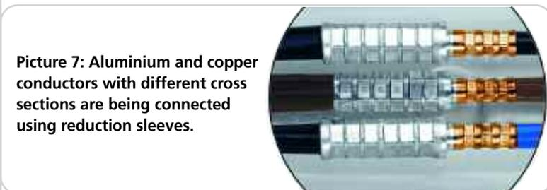
Picture 7: Aluminium and copper conductors with different cross sections are being connected using reduction sleeves.
